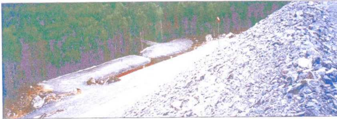
Figure 3.22: Ditch for collection and flow measuring of seepage water alongside the dam [66, Base metals group, 2002]
