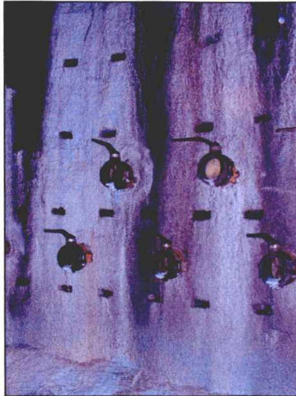
Figure 4.21: Backfill drainage system
