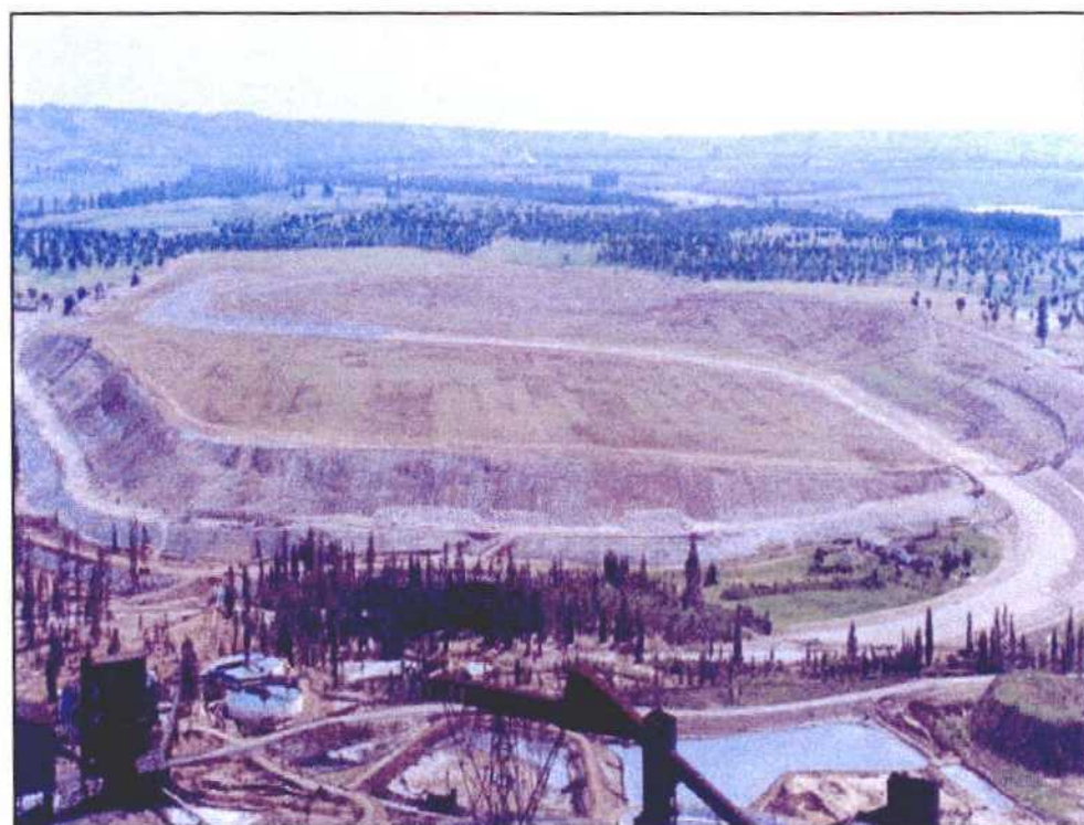
Figure 4.6: Collection and discharge channel at closed Apirsa tailings pond
