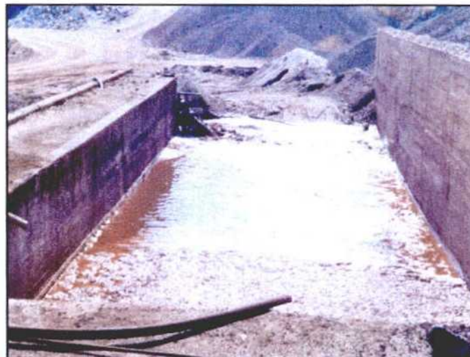
Figure 1.24: Example of a small tailings settling basin
