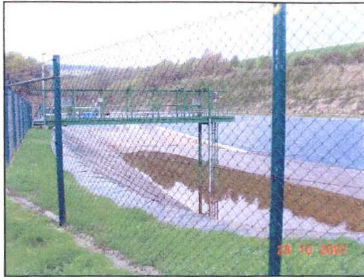
Figure 3.74: Water retention basin of German potash mine
