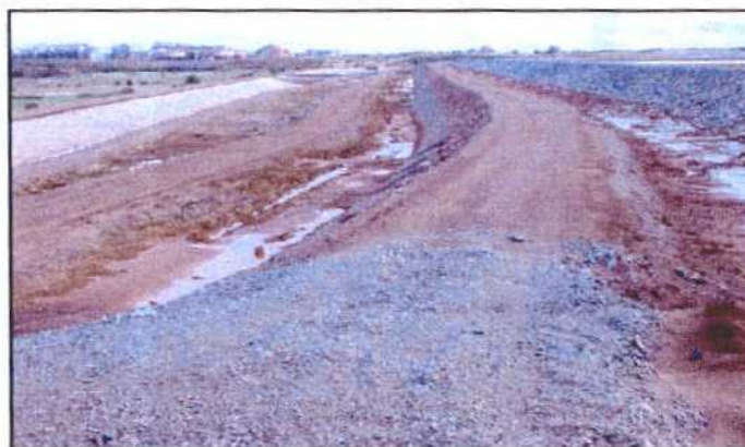
Figure 2.40: Dams raised using the upstream method at the Aughinish site
