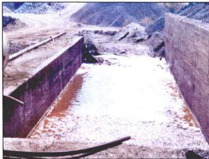
Figure 3.49: Dewatering of tailings in concrete basins [110, IGME, 2002]
