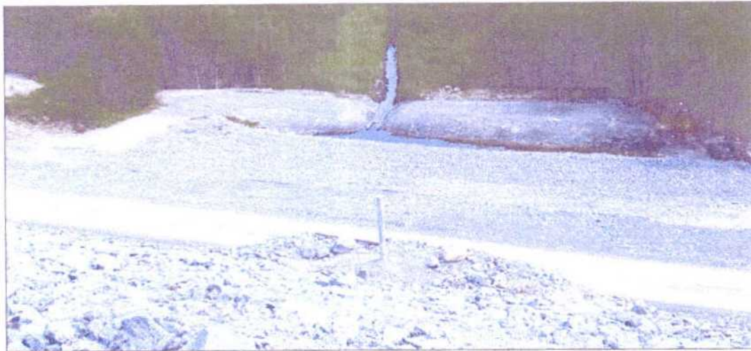
Figure 3.23: Another ditch for collection and flow measuring of seepage water alongside the dam [66, Base metals group, 2002]
